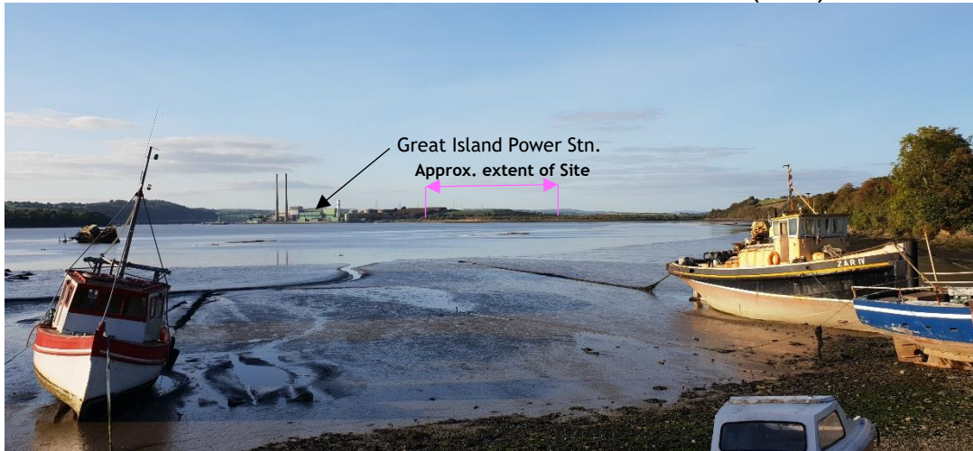
Photo 11.1 Waterford Harbour to Great Island from the southeast (Nook)
