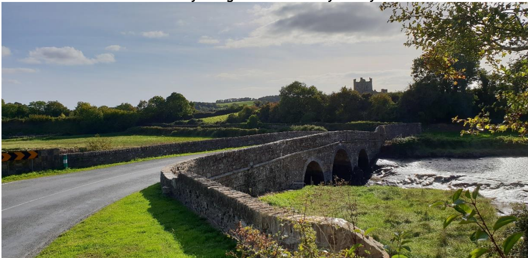
Photo 11.10 - View of Dunbrody Bridge with Dunbrody Abbey in distance
